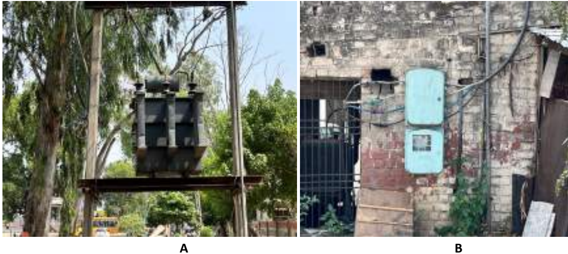
A - 100 KVA POLE MOUNTED TRANSFORMER INSTALLED FOR THE CAMPUS
