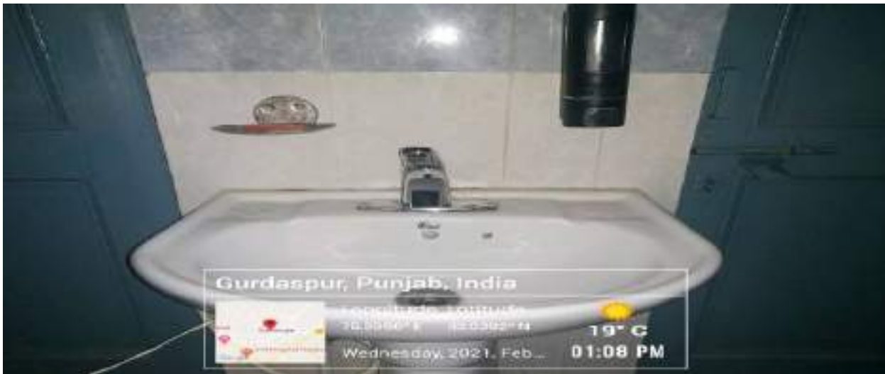
Fig: Sensor based wash basin Taps being used in building of PT.MLSDC Gurdaspur
