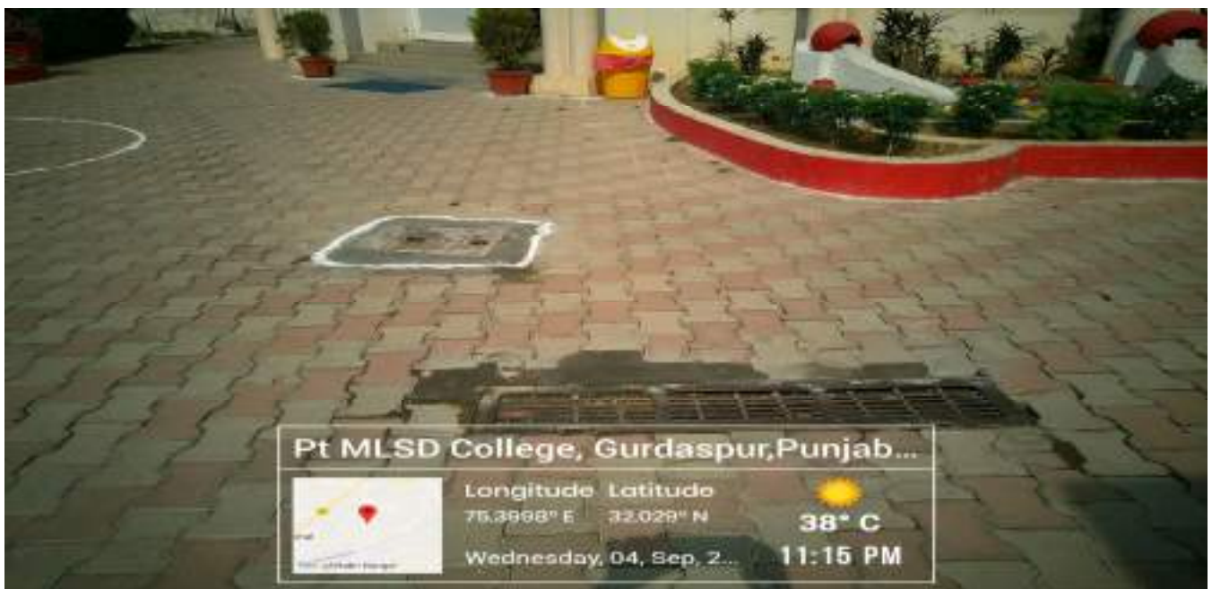
Inlets for Rainwater charging wells
