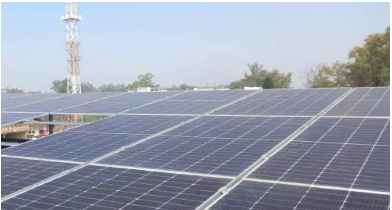
A Rooftop Solar Power Plant of Capacity 20 KWP installed in Campus
