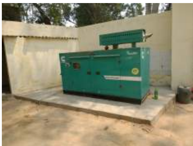
Existing DG Set 62.5 KVA installed in the college
